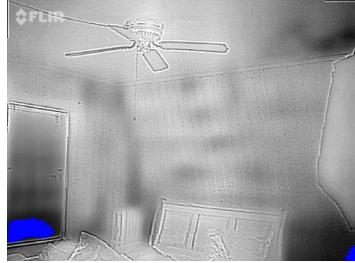
Heat map of the room, illustrates where losses are occurring. Dark areas indicate where heat is escaping.
