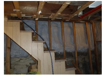
Basements air sealing in floor joists, around pipes to outdoor walls, and more.
