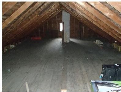
Attic insulation below the floor keeps heat from escaping through the roof.
